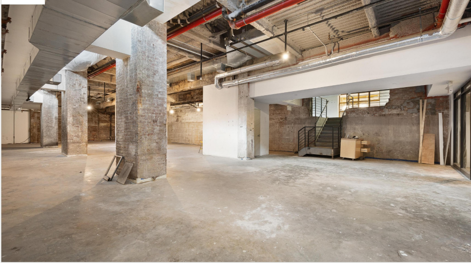
EXPOSED BRICK COLUMNS
